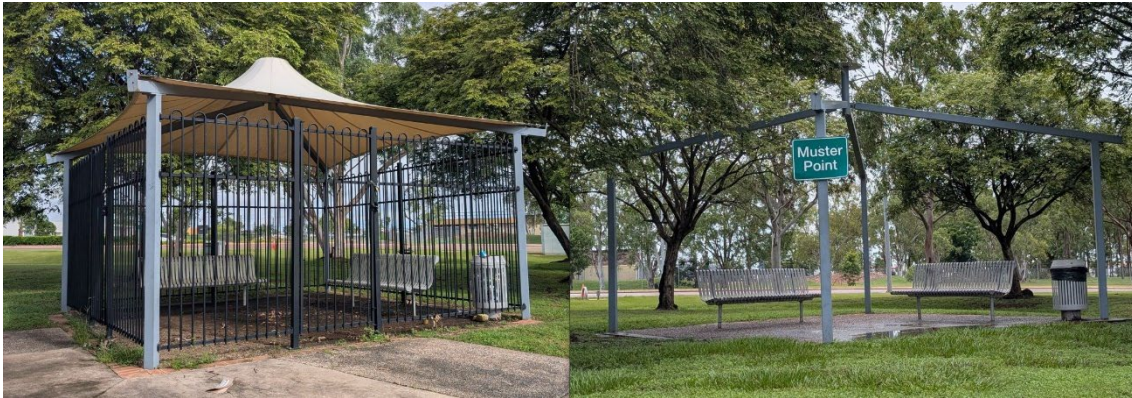
Figure 4. Benches locked up and shade cloth removed, Palmerston GP Super Clinic
