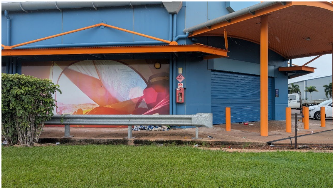
Figure 18. Vacant property provides temporary shelter for rough sleepers
